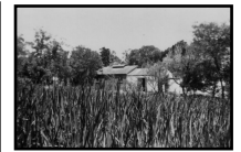
Carpentary shop (early C19)
