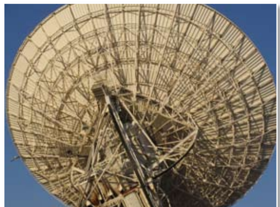
Side view (top) and close-up (above) of the former NASA deep space tracking station, converted and upgraded as the HarRAO 26-m dish for radio astronomy.
