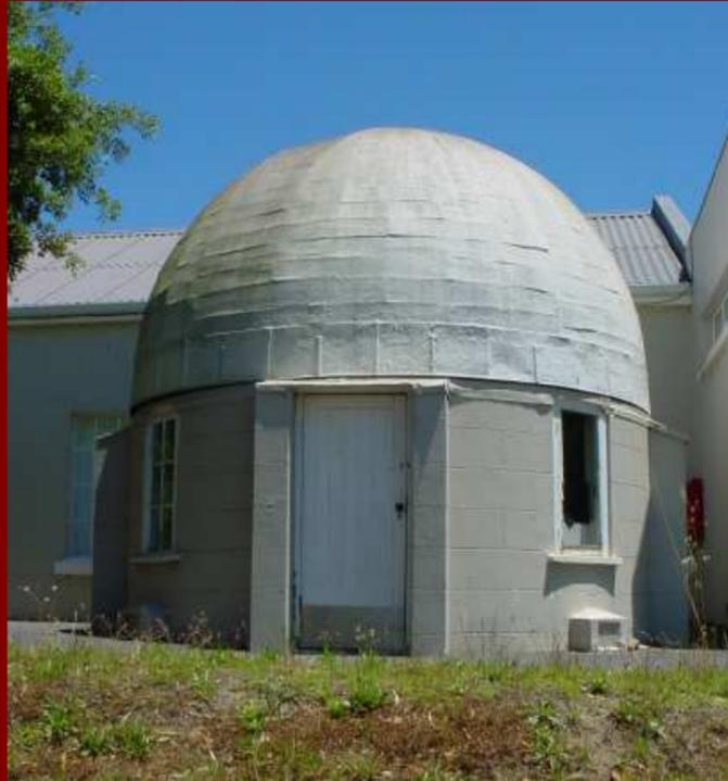
The DOME, pre-fabricated in England, is the oldest one on the site and was built in 1849 when Sir Thomas Maclear was HM Astronomer. It runs on cannon balls. At first it housed a 7-inch telescope by Merz of Munich (now attached to the 18-inch reflector elsewhere on site). The original Merz mounting was replaced by a Troughton and Simms one in 1874, probably that at present in the dome.
