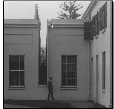
The Transit and the Mural Circle could only move along the north-south direction (called the Meridian). Shutters or 'chases' in the Main Building opened to allow the telescopes to see out. The end of the Airy Transit Circle can just be seen.
