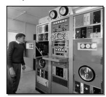
In the second half of the 20<sup>th</sup> century, the Observatory's clocks (above) were based on quartz crystal oscillators and were checked by radio signals from the atomic clocks at the Republic Observatory in Johannesburg. The time was accurate to a few milliseconds.
