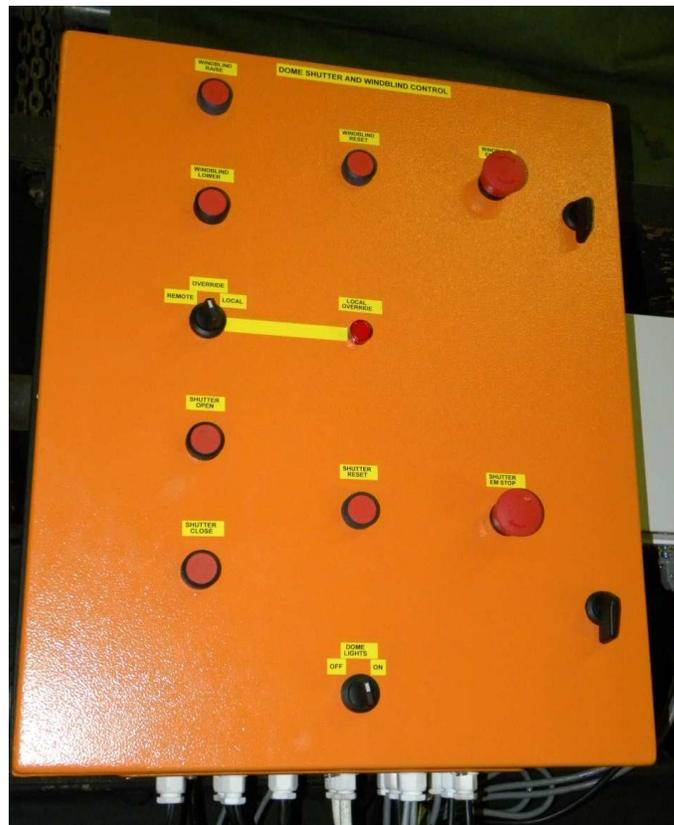
Figure 2.6: Shutters and Wind Blind control cabinet on the catwalk.
