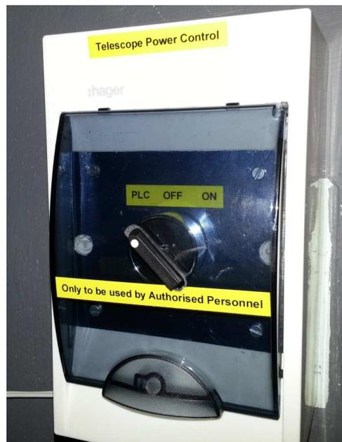
Figure 2.1: The new power switch at the top of the stairs. Ordinarily, it should be in the “PLC” position, day and night. Observers should not use this switch unless authorised by a technician.
