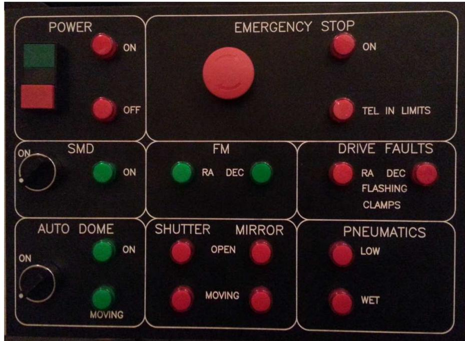
Figure 2.2: The new control panel installed in the warm room in April 2013. Power to the slow motion drive is controlled by turning the switch in the “SMD” section. When the drive power is on, the green light illuminates.
