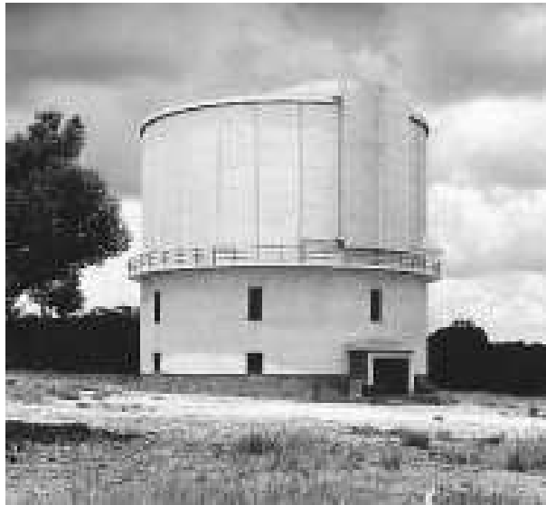
Figure 1: The turret housing the 74-inch telescope in Pretoria (photograph SAAO archives).
