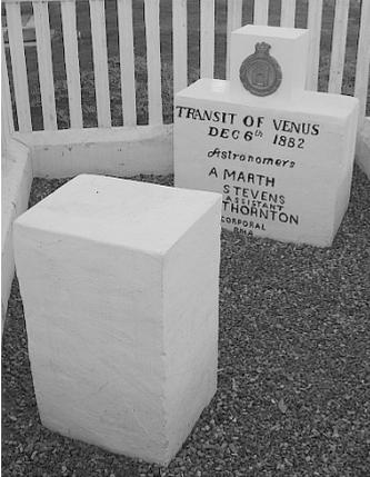
**Figure 1 (left)** The two surviving piers in Touws River. The block carrying the National Monuments plague was later added to the far (south) pier. The piers are orientated N-S with the north pier slightly higher – the opposite to a standard equatorial set-up in the southern hemisphere. (Picture: Prof George Tucker)
